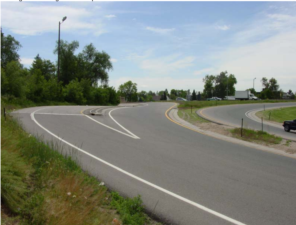
FIGURE 2 Frontage Road Merge onto Ramp
