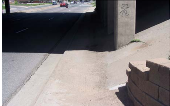
Narrow attached sidewalk under US 6 bridge (east side of Wadsworth)
