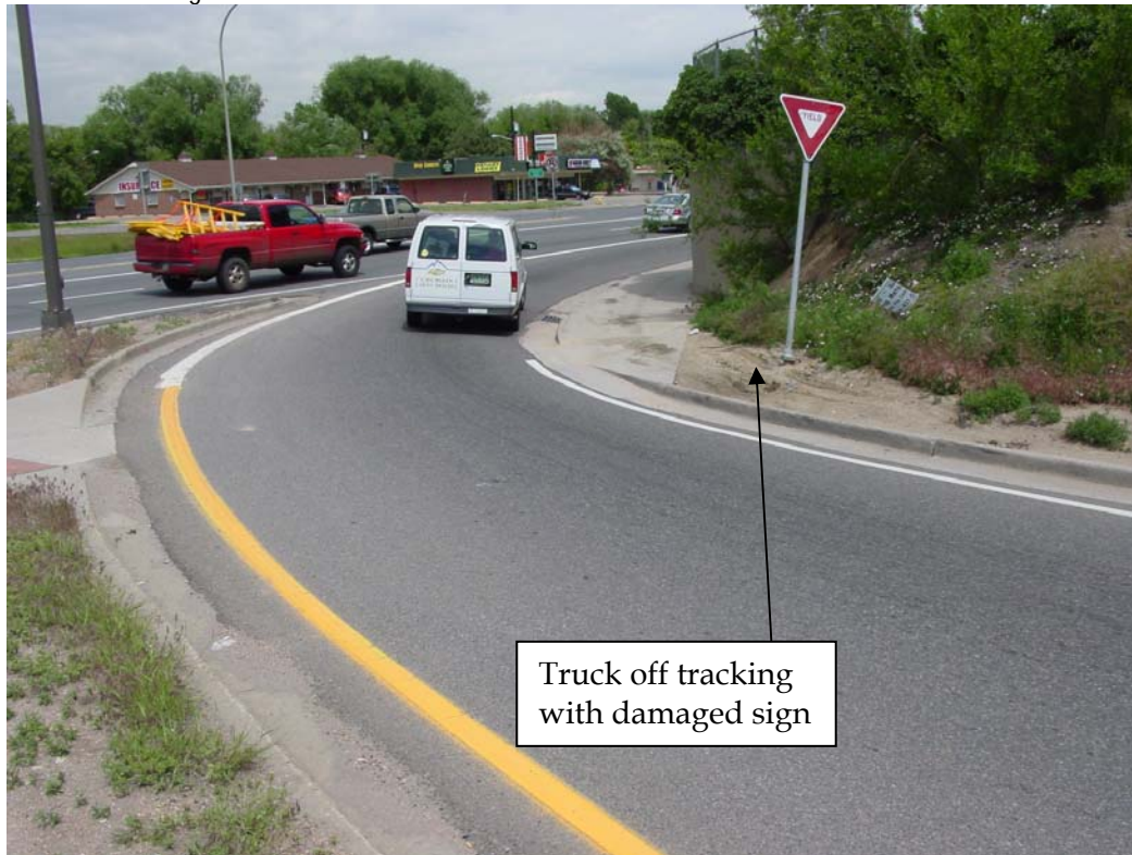
FIGURE 3 Truck Off Tracking at NE-1 Intersection
