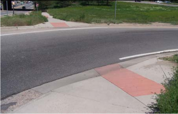
Sidewalk crossing at high-volume on-ramp (NB Wadsworth to EB US 6)
