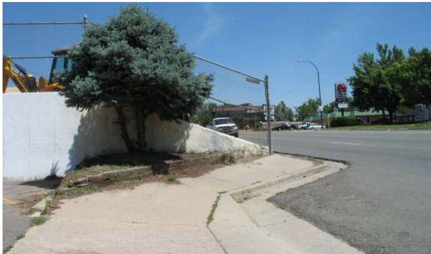
PICTURE 11: CAST-IN-PLACE WALL ON WEST SIDE OF WADSWORTH BOULEVARD, LOOKING NORTH
