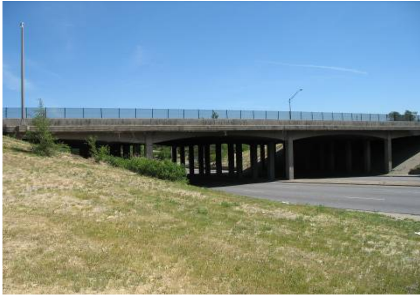
PICTURE 3: SIXTH AVENUE BRIDGE OVER WADSWORTH BOULEVARD, LOOKING NORTHEAST
