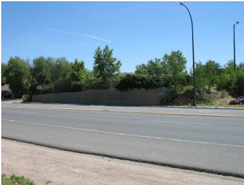
PICTURE 6: WALL AT NORTHEAST CORNER OF SIXTH AVENUE AND WADSWORTH BOULEVARD, LOOKING NORTHEAST
