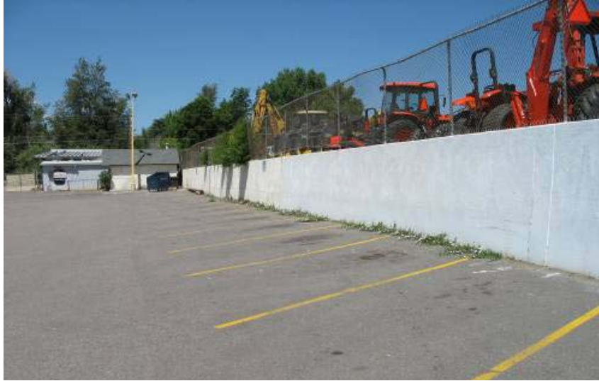
PICTURE 10: CAST-IN-PLACE WALL ON WEST SIDE OF WADSWORTH BOULEVARD, LOOKING WEST
